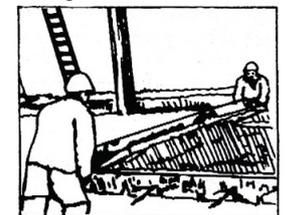
Using heavy steel straightedge or wooden float to level topping.
