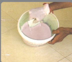
Mix Resin & Hardner together
