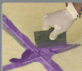
Fill joints using float
