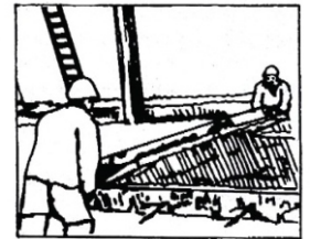
Using heavy steel straightedge or wooden float to level topping.
