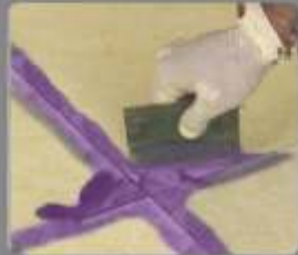
Fill joints using float
