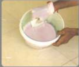
Mix Resin & Hardner together
